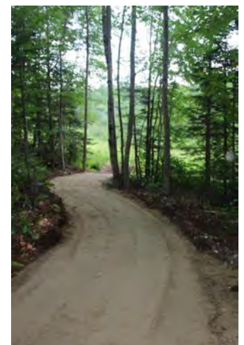
Lower section of newly constructed trail.
