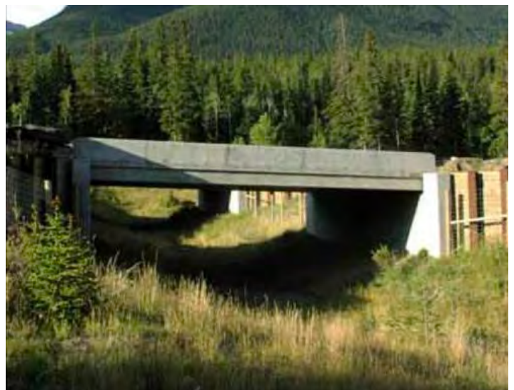
Photo top: Overhead view of the proposed location of the Farrar Farm Wildlife Crossing (shown in yellow); Photo bottom: Example of how the proposed Farrar Farm Wildlife Crossing would look.
